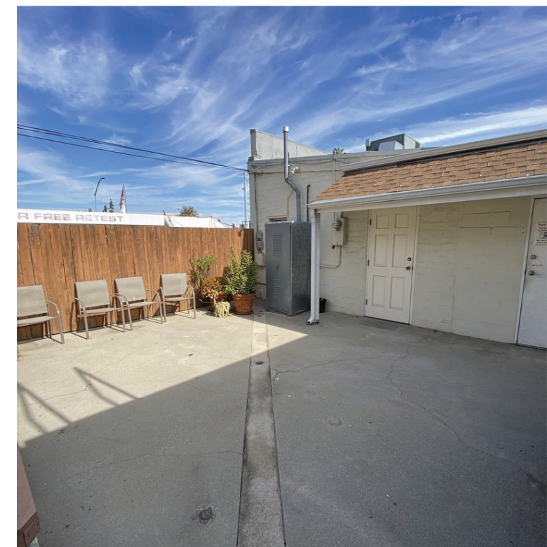
Rear Outdoor Patio (Retail/Office Building)
